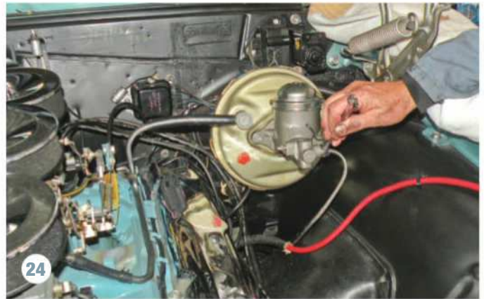
24 Here is the new master cylinder installed on the firewall. After connecting the new line, we went back through the system from connection to connection, from front to rear, and rechecked all of the fittings to make sure each one was threaded correctly and tight.
